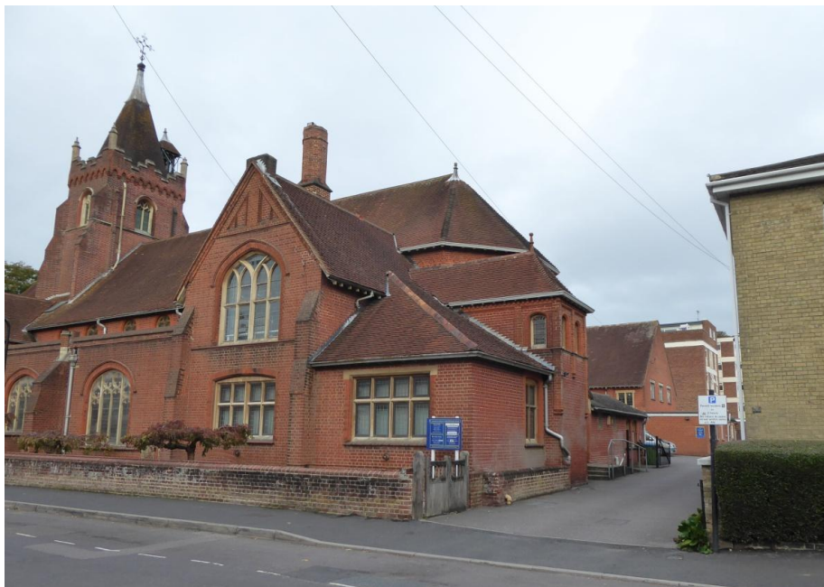
View into the site from Alma Road – halls roof in the distance
